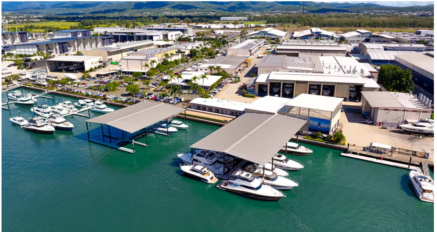
The 16.8 hectare Riviera factory at Coomera is the largest luxury motor yacht building facility in the southern hemisphere.
